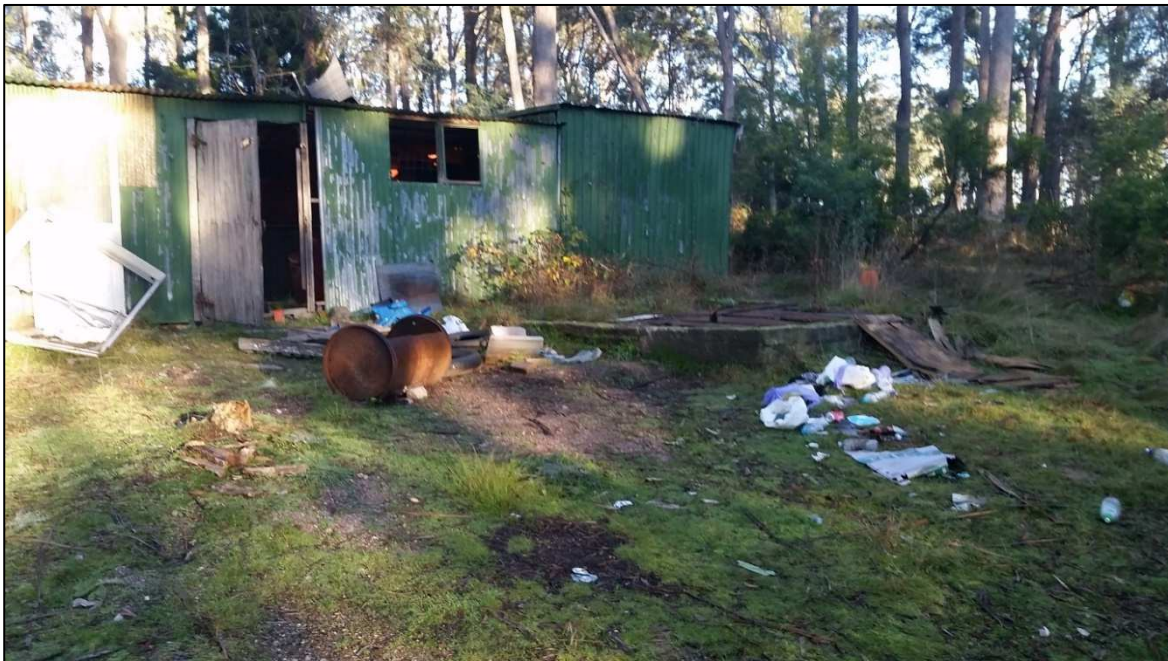
Plate 2: Corrugated iron structures and rubbish in the DAD in the south west of the proposal area
